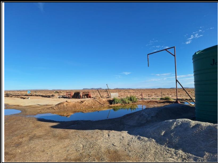
JOJO TANK AND WATER FILL STATION
